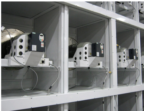
Figure 2: Altivar 212H••••S2 Drives in a SmartCube
