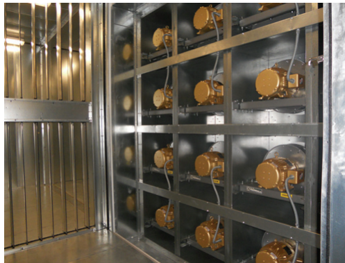
Figure 1: Multiple Fan Array
