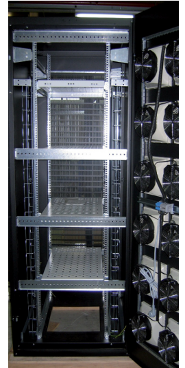
Ventilated 19" enclosure with fans mounted on the doors Enclosure dedicated to extract a lot of heat. Mainly dedicated to server application. This configuration permits to help ensuring the stability of the installation.
