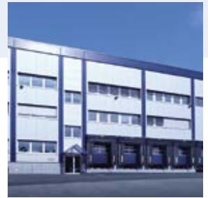
Startup of the new central warehouse in 2013
